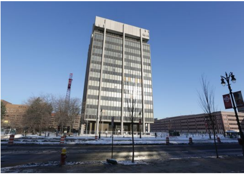
The Professional Plaza building, 3800 Woodward, also known as the Hammer and Nail building for the iconic neon sign atop the building. (Photo: Detroit Free Press)
